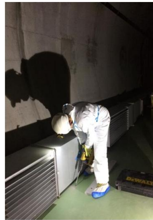
Sampling of concrete
