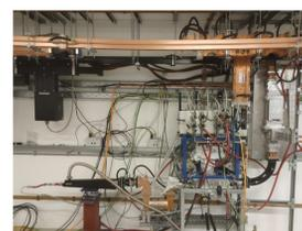
SLED Installed in Linac.
